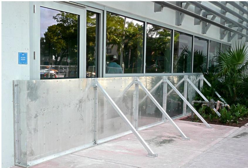
**Photograph 4.7 Temporary Flood Barrier Protecting Building Entryway**
