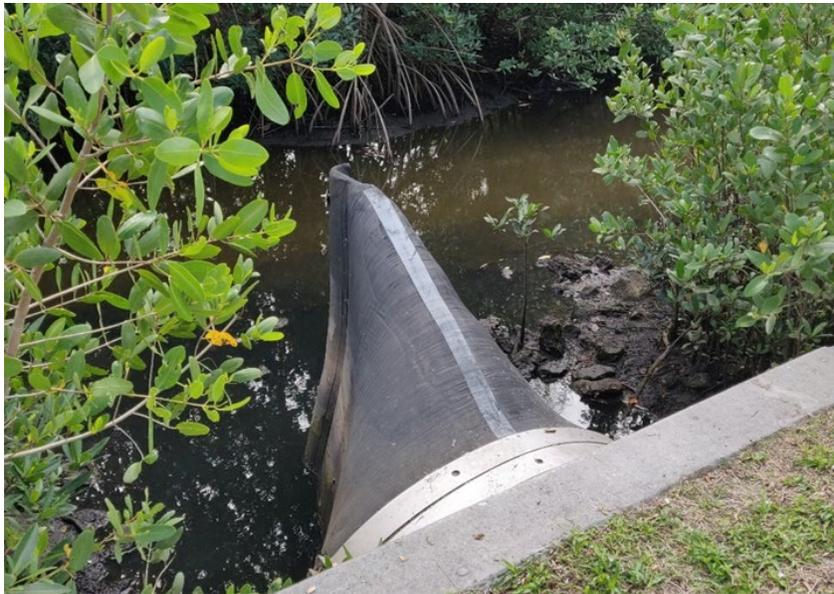
**Photograph 4.3 Stormwater Check Valve for Backflow Prevention**
