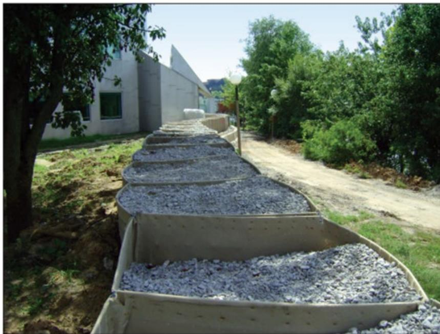
**Photograph 4.5 Gravel Filled Containers that Form a Flood Barrier**
