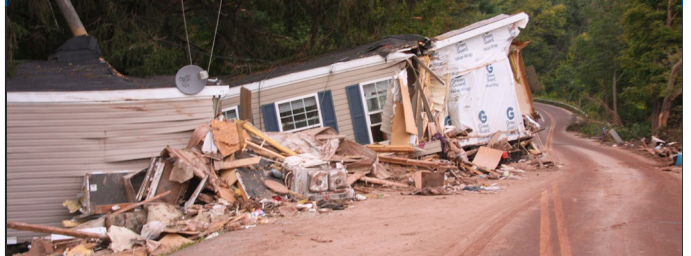
Wind Damage and Displacement of Manufactured Home
