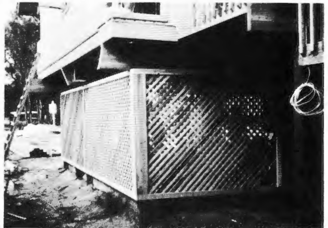
Figure 4.54. Breakaway Walls
