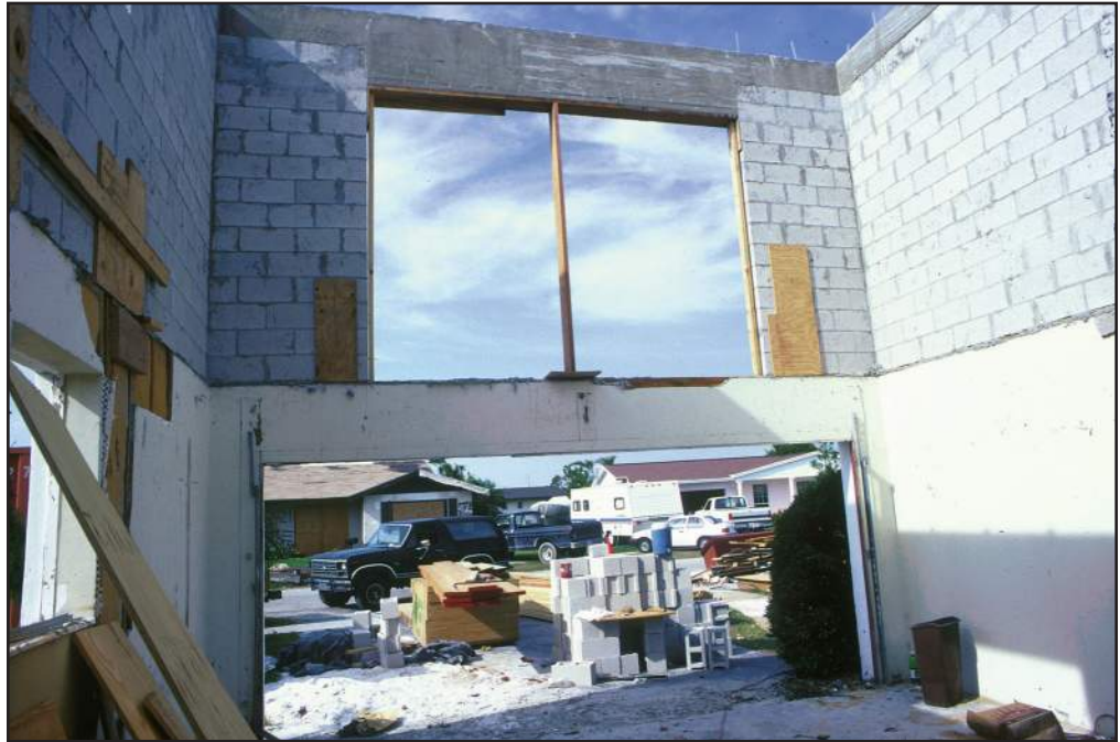
Figure 66 The new second-story walls as seen from inside the garage.
