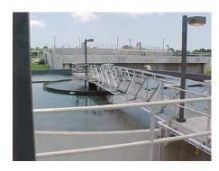
The solids in the mixed liquor settle to the bottom of the clarifier, where they are pumped back to the first anoxic basin or to the sludge holding tanks prior to dewatering and removal from the facility. The clear water then flows to the filters.
