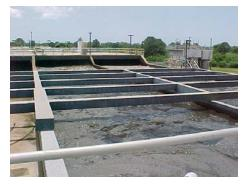
The heart of the treatment process is the aeration basin. The wastewater is mixed and aerated, providing an environment that is ideal for bacteria utilized for reducing the strength of the wastewater which is measured as biochemical oxygen demand (BOD).
