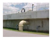
After the second anoxic stage, the mixed liquor is re-aerated to increase dissolved oxygen prior to final settling in the clarifiers.
