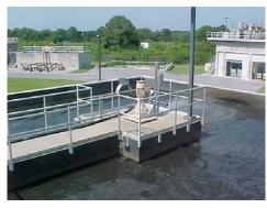
The flow continues to the first anoxic basins. This treatment step provides conditions ideal for the growth of bacteria necessary to remove nitrogen compounds from the wastewater, as required by the facility's Permit.
