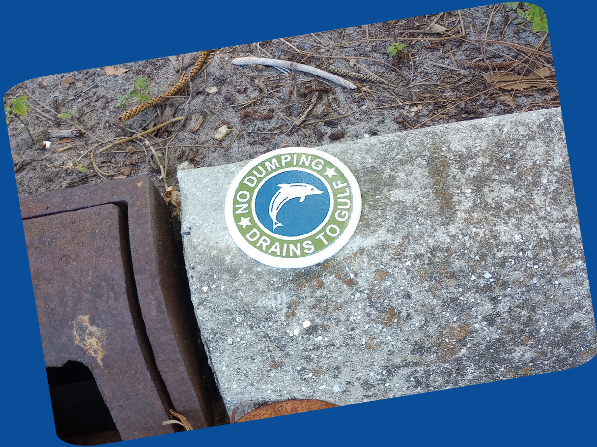
StormWater Inlet Marker
