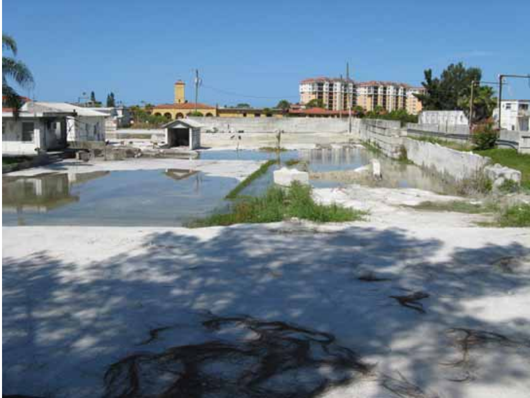
Buildings and cement that was removed, future natural landscaping
