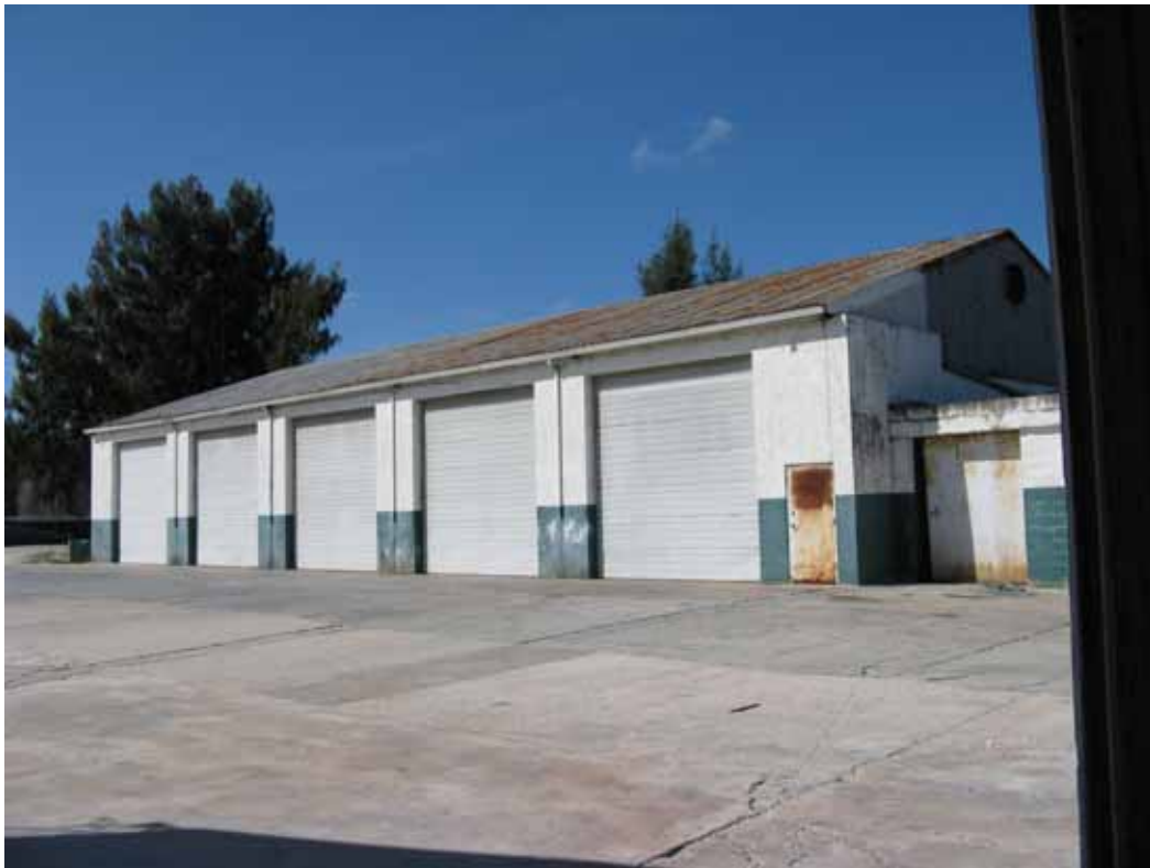
Garage building demolished
