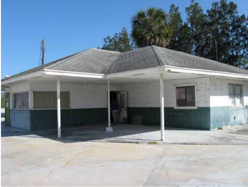
Office building that has been demolished
