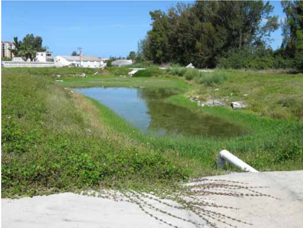
Stormwater pond that will be cleaned up and restored
