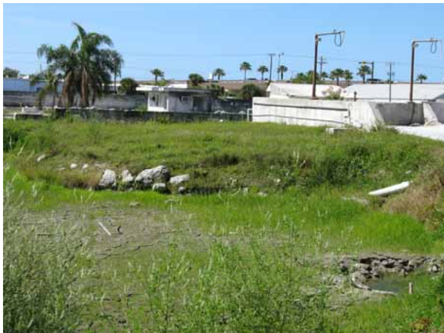
Stormwater pond to be restored
