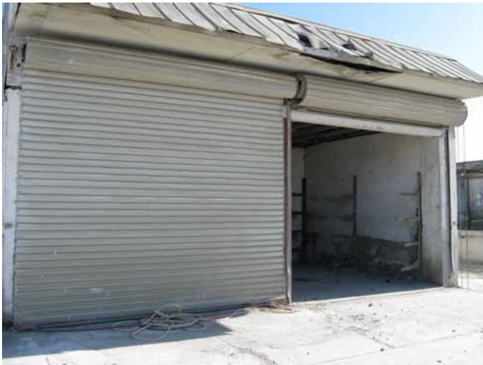
Garage building demolished
