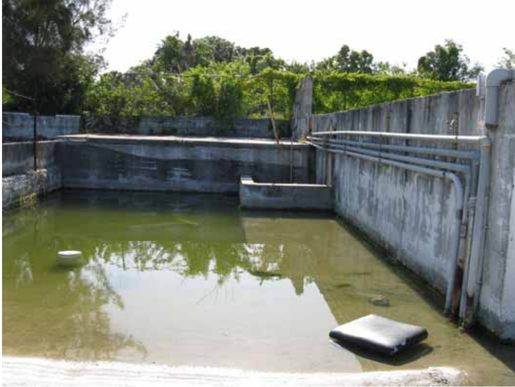
Cement area removed, future natural landscaping and trail area
