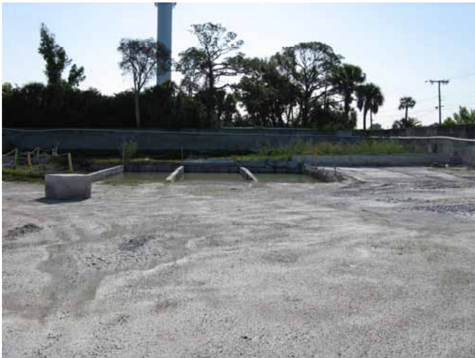
Cement area removed, future natural landscaping
