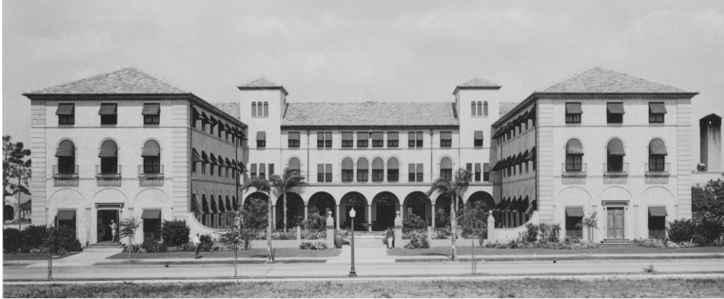
Hotel Venice, 200 Nassau St, built in 1926. Strict symmetry has been maintained while breaking the mass into three sections. The light color reflected infrared from sunlight and the awnings provided shade. The north-facing windows (not impacted by the sun) sported awnings for design consistency.
