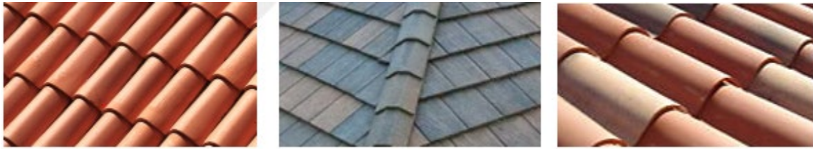
Figure 7.10.5. Permitted Roof Materials (From Left to Right: Clay, terracotta, Barrel Tiles) and Roof Photos
