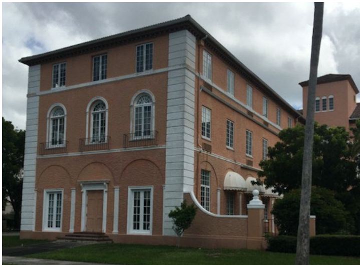
Later incarnations of the Hotel Venice, as in the left, darkened the wall color, thus providing a greater contrast with the accents. In this image, the eye is drawn toward the edges, rather than the façade as a whole. It is important to recall that the VHP stressed an integral building design rather than an assembly of parts.
